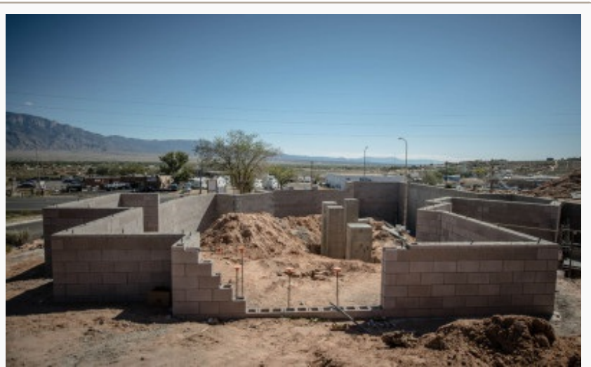
The future home of Wealth Management at Quantum and N.M. 528 being built by Rachel Matthew Development. The building is one of more than a dozen commercial projects permitted since an impact fee moratorium took effect in September 2012. (Roberto E. Rosales/Albuquerque Journal)
